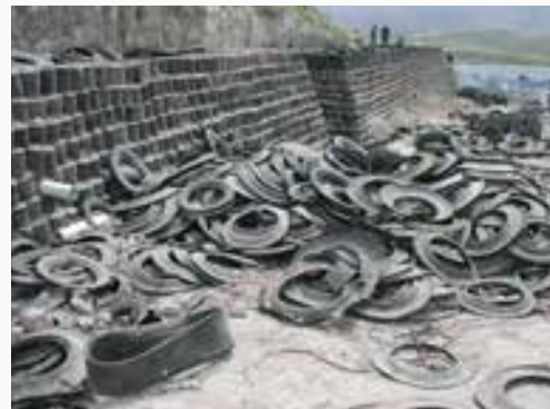
Autobanden gerecycled tot steunmuur in Tijuana
